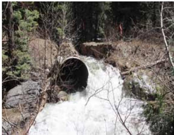
Flathead NF photo of a 4' plugged culvert putting the Emery Creek Road into trout habitat!
