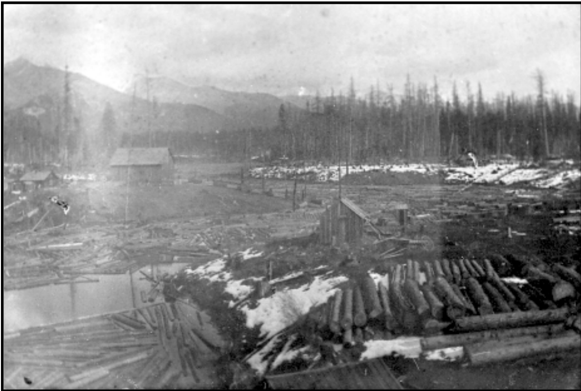
Jessup Mill Pond during peak of mill operation.
